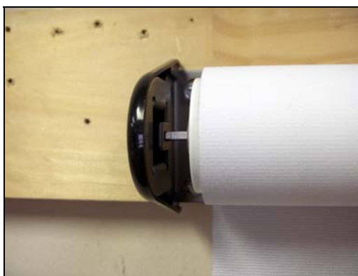
Figure 4 Setting spring end in the bracket
