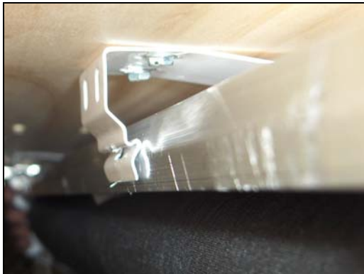
Figure 7 Cassette bracket unclipped
